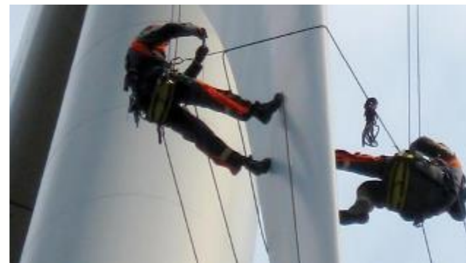
Rope access inspections are typical
