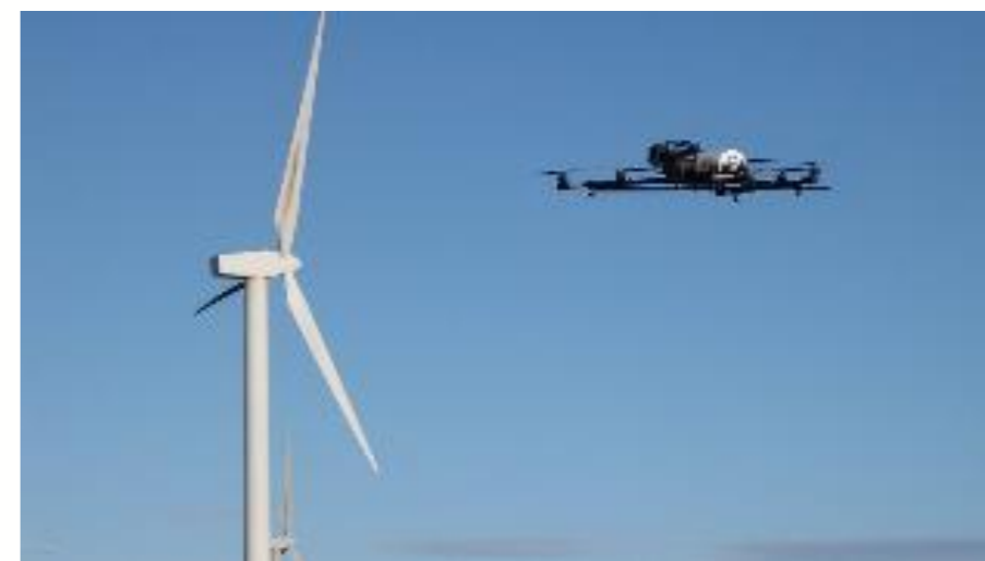
UAV blade inspections are being used
